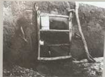
The use of an upper pivot to hang a door was suggested to the expedition team by modern examples in a village near Kermanshah, Iran.
